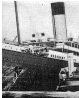
The damage below the waterline however, was said to be far more serious, also the super structure had warped. The damage is shown in the photo below, it was taken after RMS Olympic had limped into the docks in
